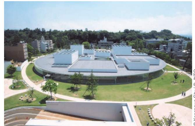
The SANAA-designed 21st Century Museum of Contemporary Art is a major attraction in Kanazawa City
